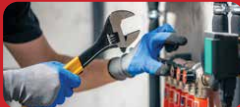
Equipment repair and replacement
