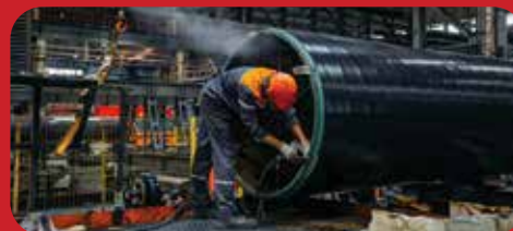
Installation of industrial equipment and technical assistance
